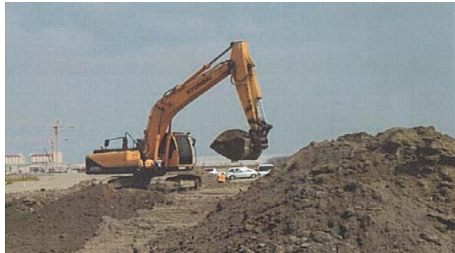
Figure 3: Construction of Road with Consolation Soil
